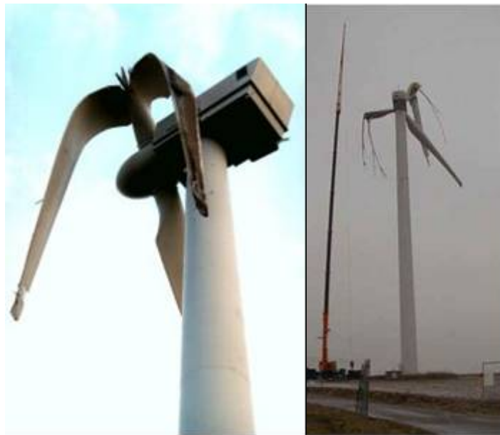
Fig. 2.2: Two examples of turbines that failed, but caused no danger to their surroundings.
